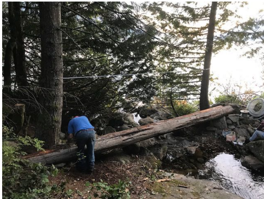
Bridge logs and wire handrail in place
